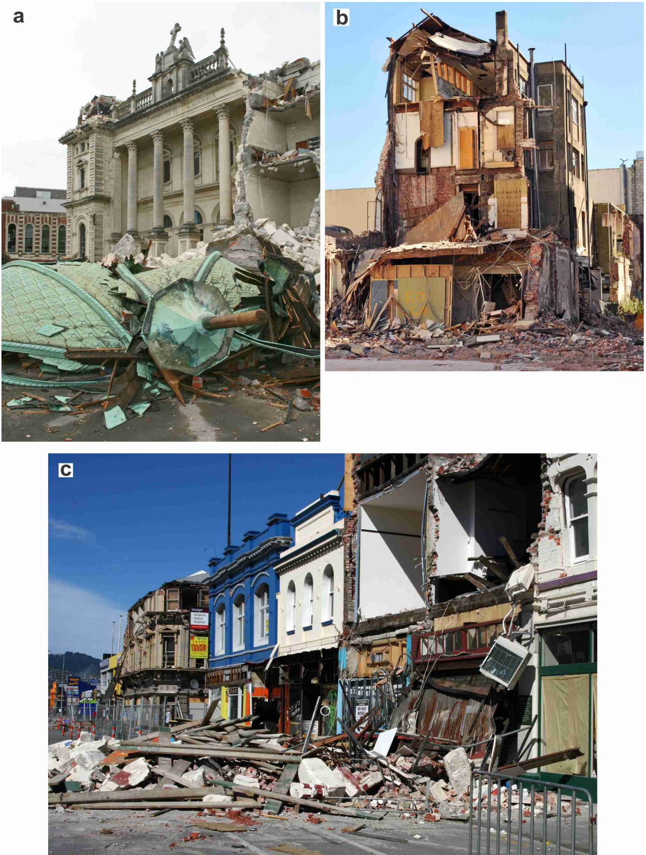
Figure 8.10: (a) Damage to the Cathedral of the Blessed Sacrament, photographer Margaret Low, copyright GNS Science, VML ID 6128. (b) Damaged building, photographer Margaret Low, copyright GNS Science, VML ID 101912. (c) Building damage in the Christchurch central business district, photographer Margaret Low, copyright GNS Science, VML ID 101881.
